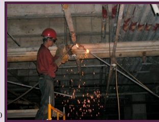
Welding in the basement
