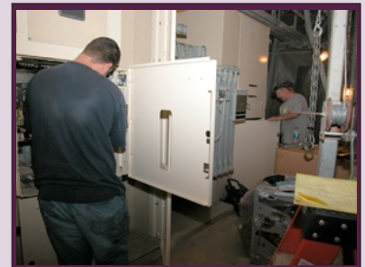
Electricians at work
