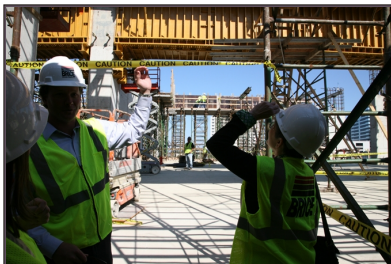
at the LCRC construction site
